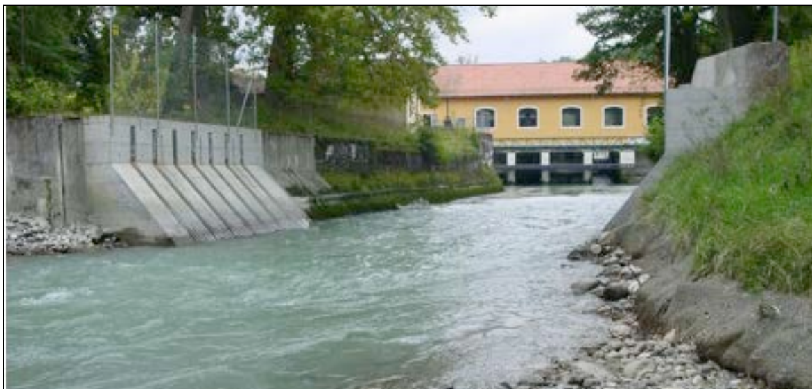
Figure 4. The tailrace electrical deterrence array at the Vessy (Switzerland) hydroelectric power plant. A series of seven electrode cables can be seen housed within the special, non-conductive concrete slab that was installed to run across the river bottom from left to right bank, thus providing full deterrence capabilities across the entire stream without being affected by floating debris. The barrier successfully deterred fish from moving upstream from the River Arve into the tailrace and powerhouse.
